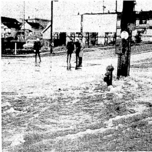
DELUGE: Water gushed from a broken main at Third Avenue North and flowed into Mercer Street this morning as police diverted traffic from the flooded intersection. A utility pole, a police call-
